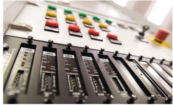
A detail of Local Control Cubicle
